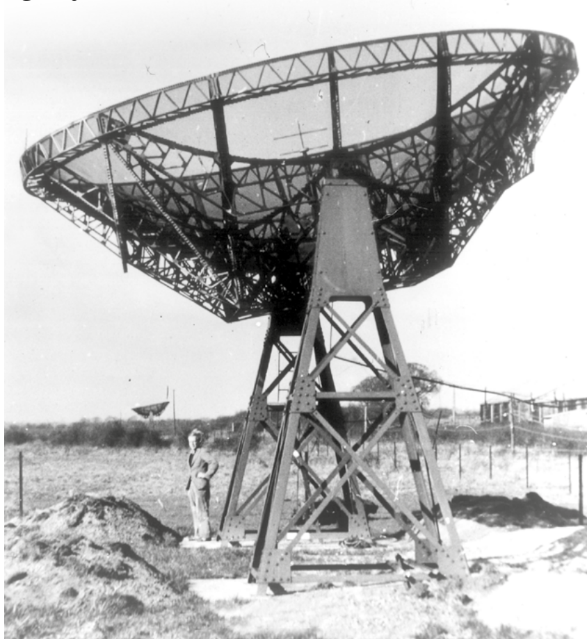
Graham Smith with the interferometer which used the two Würzburg antennae in about 1950.
