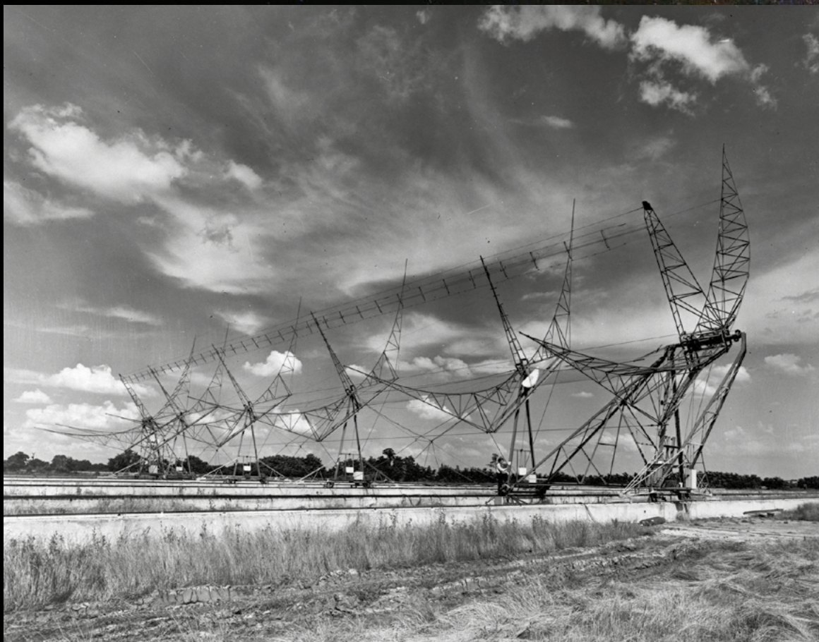
Moving element of the 4C interferometer.
