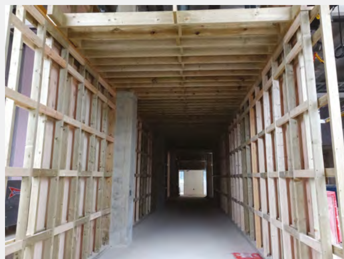
TOP: Office corridor in Wing 3 level 2. BOTTOM: Cryostat timber partitions in Wing 1 level 0.
