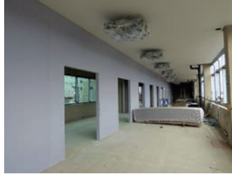
Fig. 3. First fix Mechanical, Electrical and Plumbing (MEP) and partitions in wing 4.
