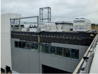
Fig. 1. Chillers on the roof.
