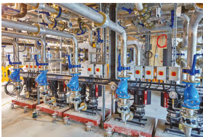
FIG. 4. Part of the GSHP plant room.
